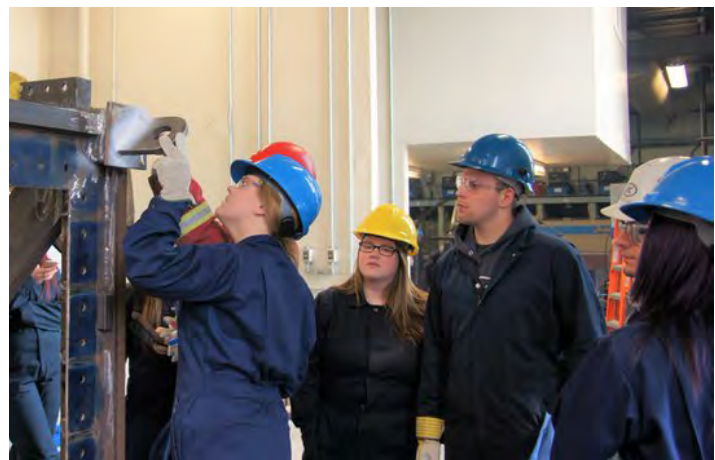
Students performing QA/QC on critical welds during construction of WERC pump
