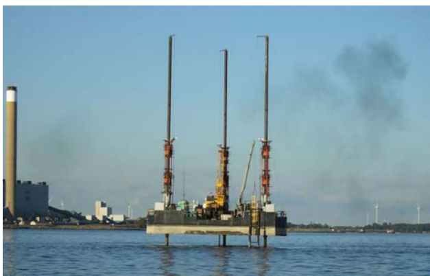
Geotechnical Drilling.
